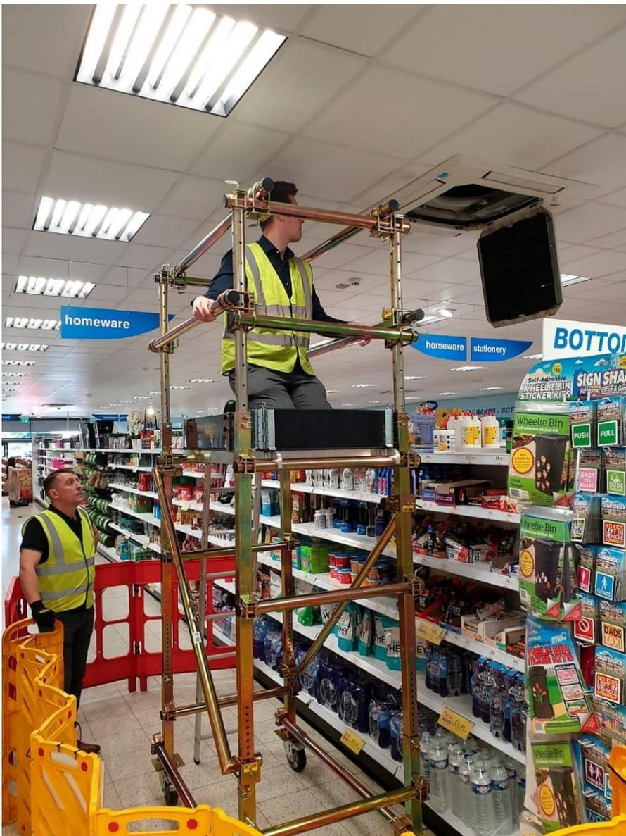
Real time overnight maintenance issues exist as time constraints increase labour costs, with safety being a key component. The strategic use of the LOBO System to gain rapid access for working at height issues may in part alleviate these issues.
