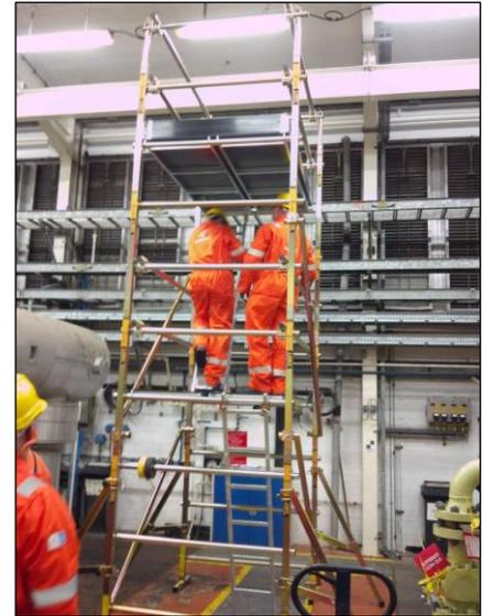
No problems apart from the recurring issue of WAH controls during the transition of placing the guard rail on from the seated/kneeling position when the boards are placed. A discussion was held with the team and this can be alleviated by using an advanced guard rail.
