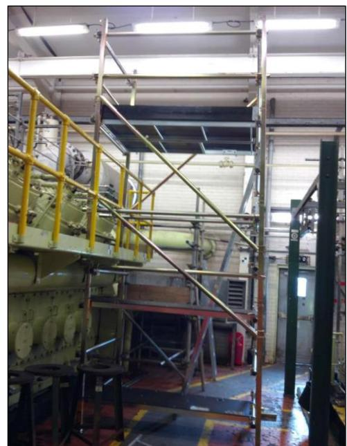
Some minor problems with getting around the obstruction of the guard rail on the gantry, which was eventually overcome by the demo team. Initially I was concerned about the stability, but after climbing the ladders to the top lift I discovered it was no more unstable than a tube and fitting tower of the same size. There is also an option to use longer stabilizers/outriggers to provide added stability.
