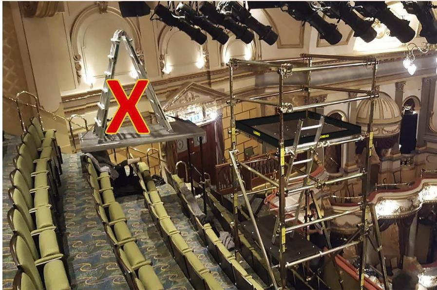
The LOBO System comprises of trestle legs that vary in size, and adjustable extensions with fixed side clamps. Steel tubes can then be passed through the clamps, which are hand tightened to form a structure to suit the application. Sway braces, toe boards, wheels, handrails, out riggers and a lifting beam
