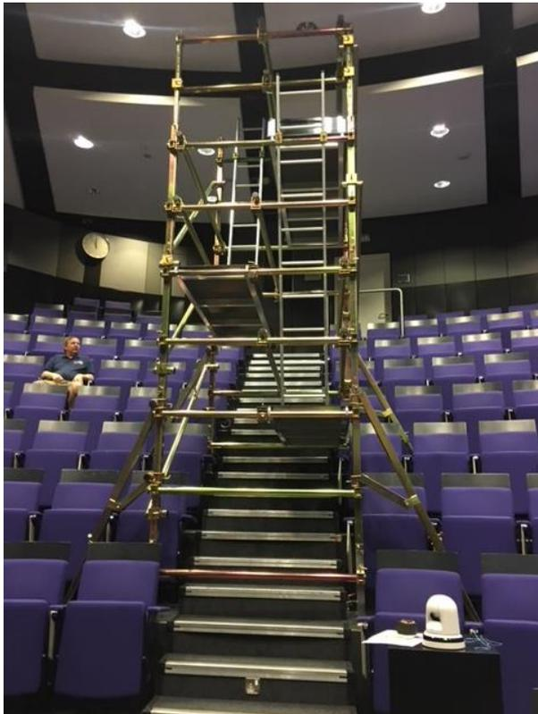
Access equipment which is unstable or rickety, which does not fit properly and is therefore dangerous, should never be used.
