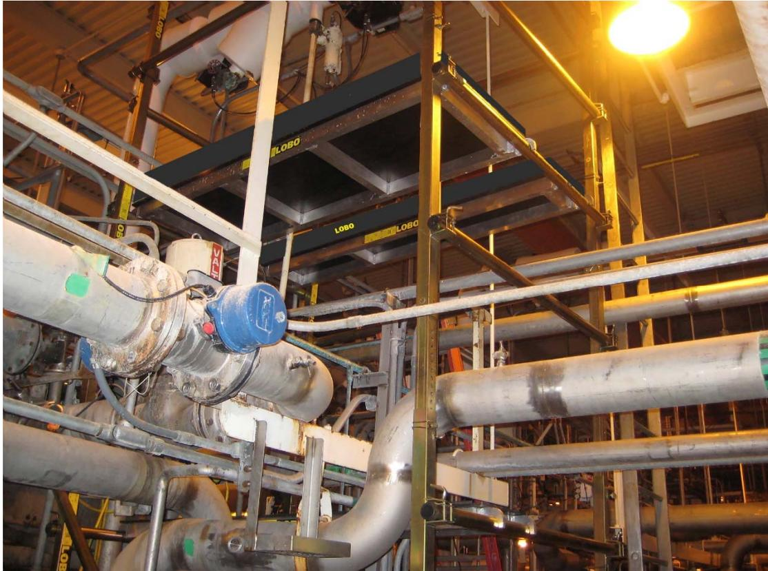
Your own in-house maintenance crews can assemble the LOBO System quickly, easily and safely around, under or above machinery or conveyors. To ensure safety, handrails can be fitted in seconds, at any point in the system, and at any stage of the assembly process. Staff should never be exposed to the risk of a fall.
