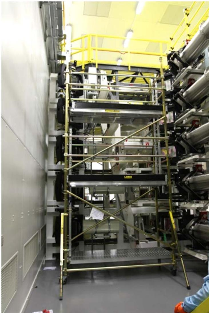
The system can be assembled, disassembled and reassembled quickly and is immediately available, unlike traditional scaffolding that must be assembled by qualified scaffolders.
