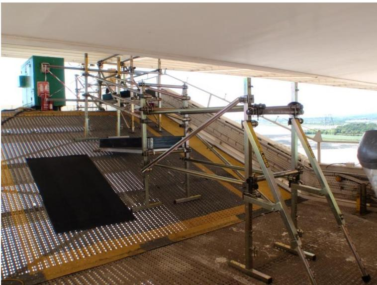
assembled by anyone, as the components are modular. LOBO's electroplated steel legs and components can be flat packed when not in use and transported easily, for storage or utilisation elsewhere, especially suitable for restricted entry points.
