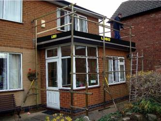
Outriggers are used to stabilise the legs & the ladder is secured using LOBO ladder clamps. LOBO Systems' no tools assembly feature means it can be constructed around any flat roof or surface in minutes and flat packs for easy transport.
