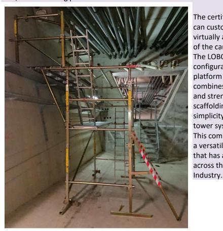
The certified LOBO user can custom assemble virtually any size or shape of the cantilever The LOBO System is a reconfigurable work platform product that combines the flexibility and strength of traditional scaffolding with the simplicity and mobility of tower systems. This combination provides a versatile access system that has applications right across the maintenance
